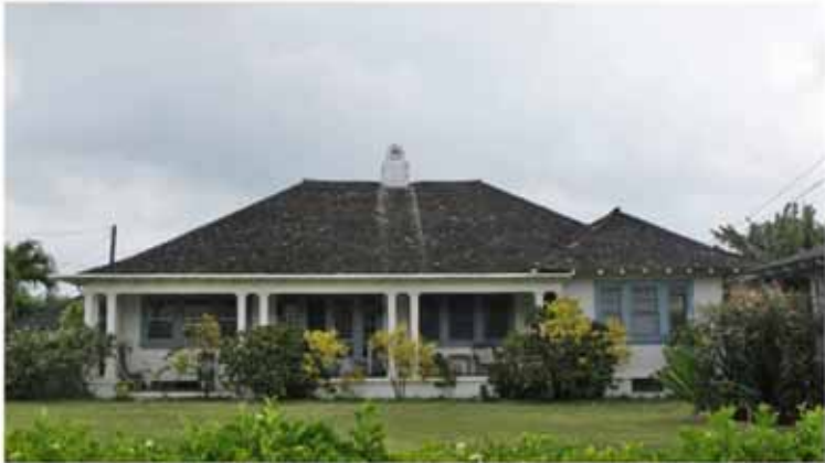
Single-story village house with engaged front lanai
