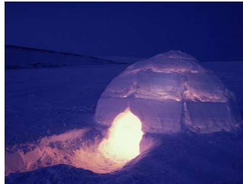
Igloo Uses Snow as Insulation
