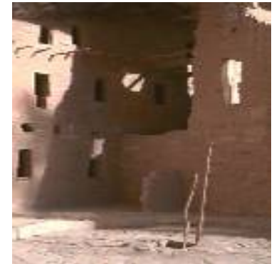
Pueblo Uses Earth for Thermal Mass
