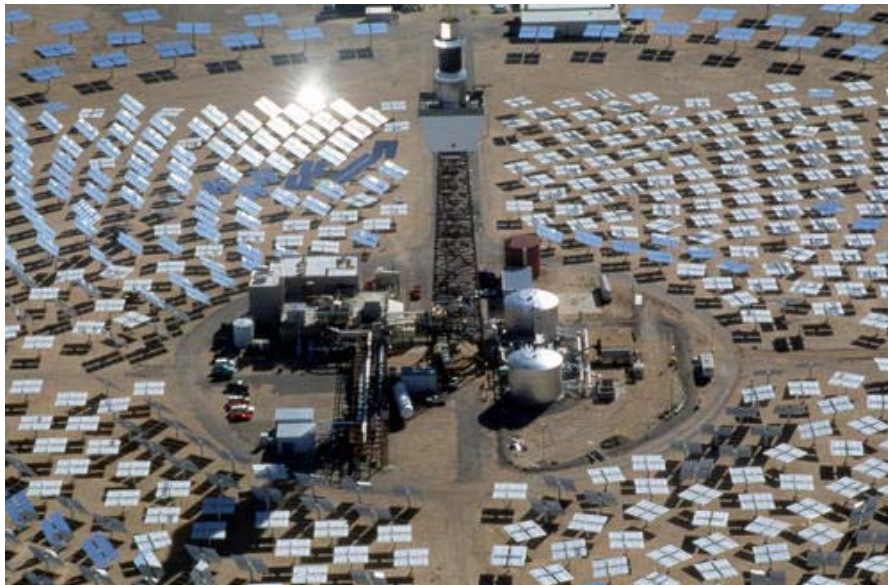
Figure 3-16. Solar Two Central Receiver Installation
