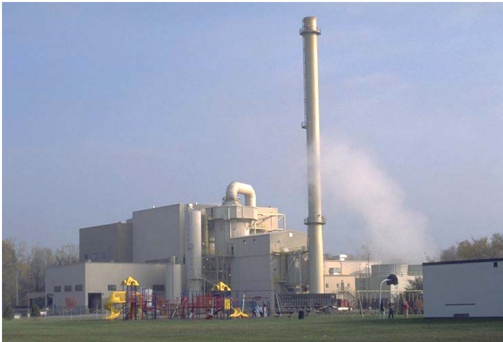
Figure 3-7. Central Wayne Waste to Energy Plant.
