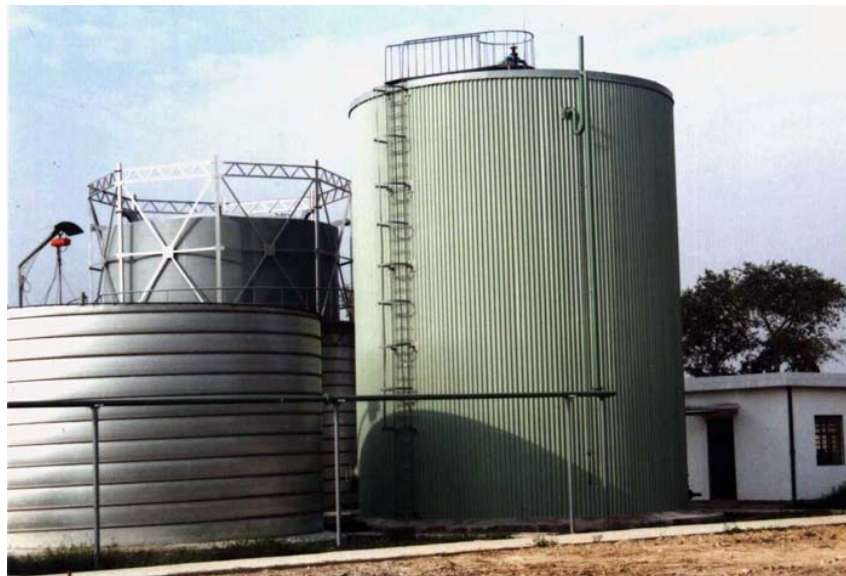
Figure 3-4. 500 m 3 Digester Treating Manure from a 10,000 Pig Farm in China. 8
