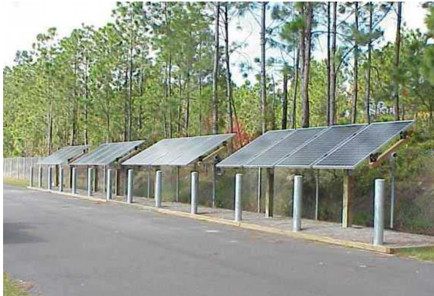
Figure 3-13. Photovoltaic Solar Panel Installation.
