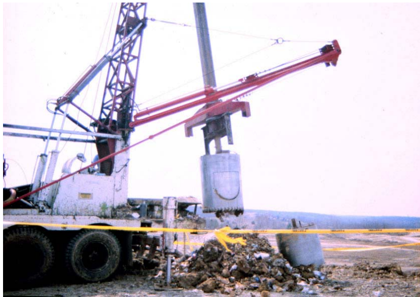
Figure 3-5. LFG Well Drilling.
