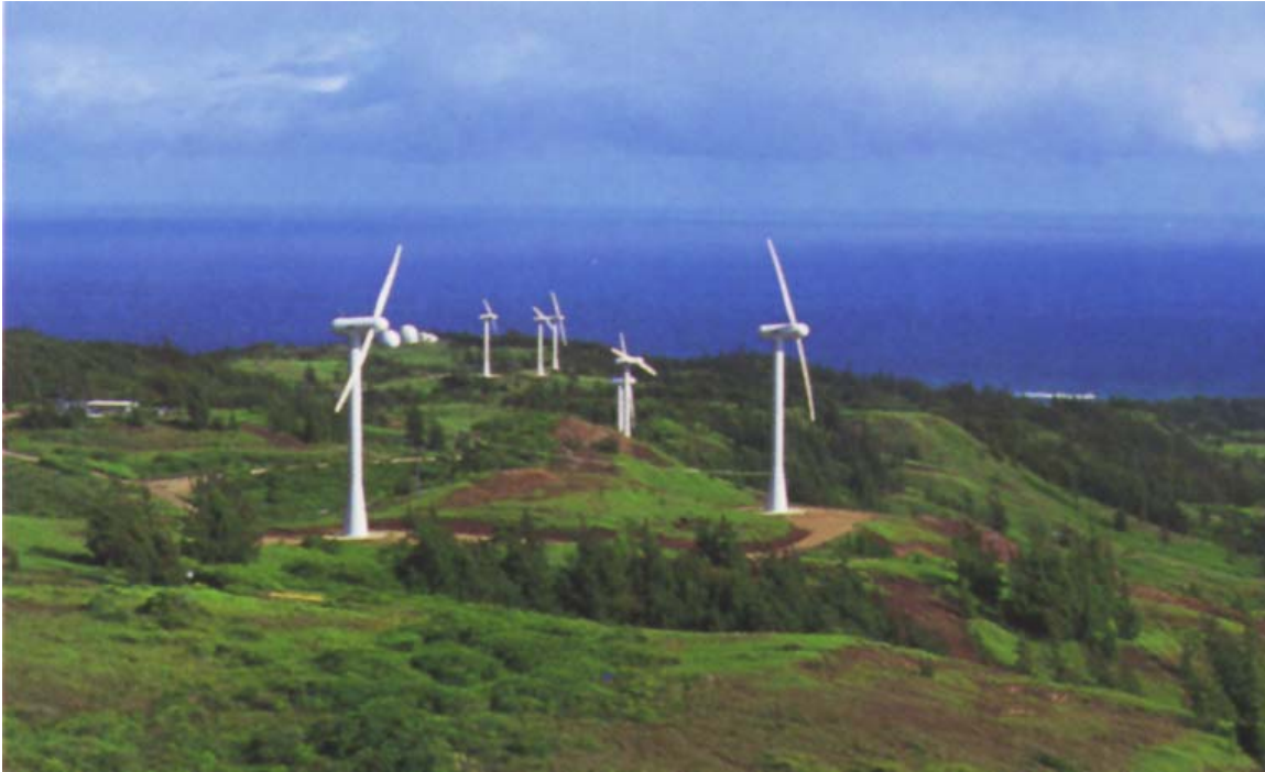
Figure 3-18. 9 MW Kahuku Wind Farm on Oahu, Now Decommissioned (Source: DBEDT).
