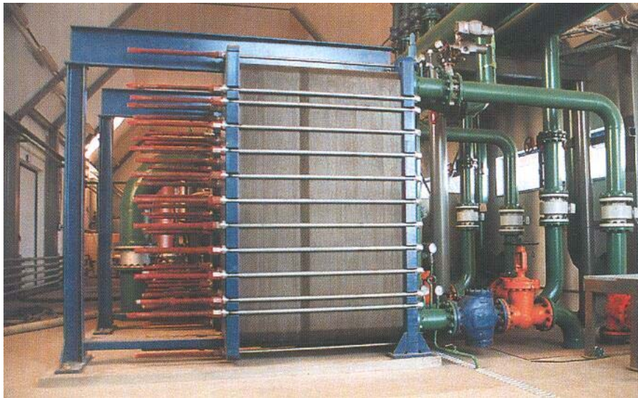
Figure 3-20. Geothermal District Heating Equipment.
