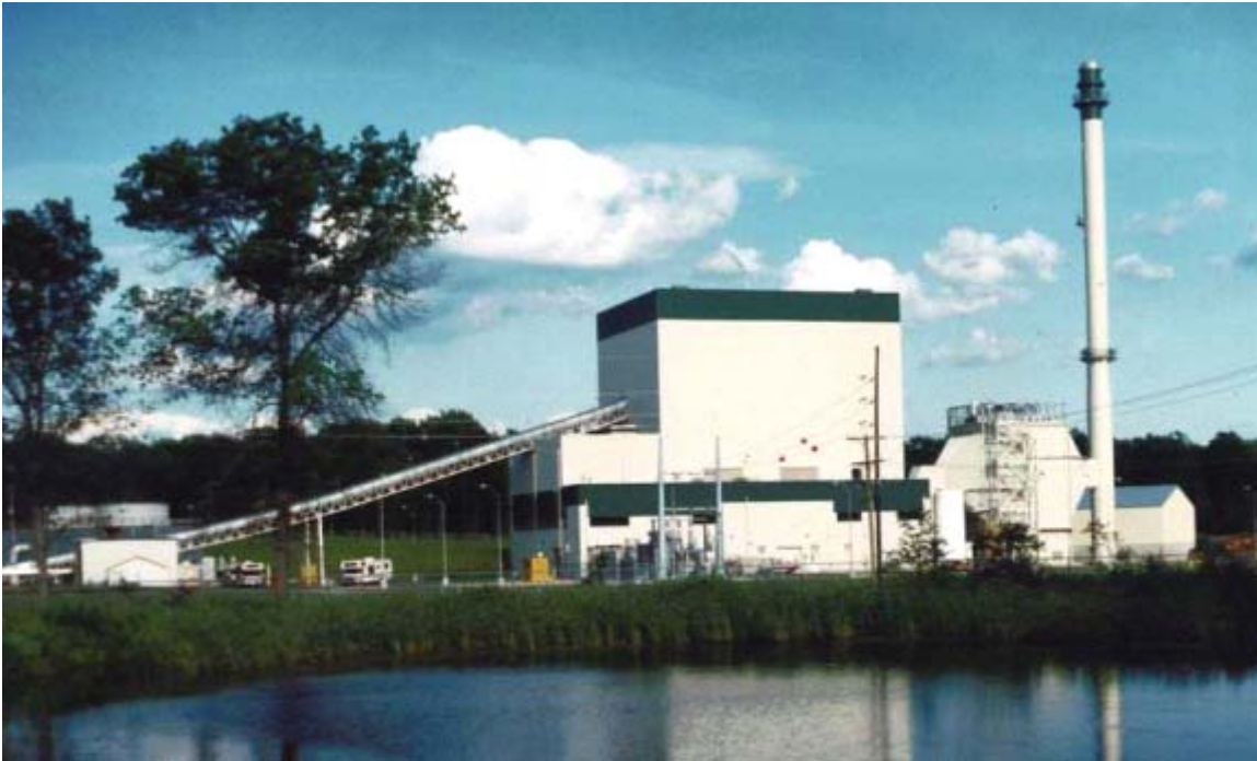
Figure 3-2. 35 MW Biomass Combustion Plant.
